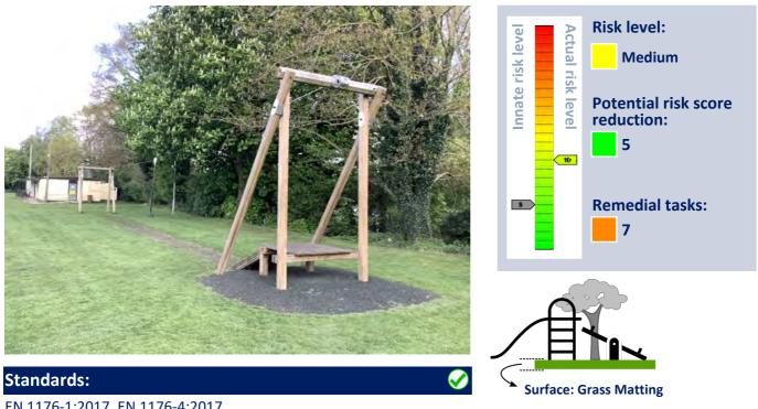
EN 1176-1:2017, EN 1176-4:2017 The item and its surfacing (where applicable) meet with the requirements of the relevant standards.
