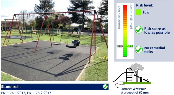
EN 1176-1:2017, EN 1176-2:2017 The item and its surfacing (where applicable) meet with the requirements of the relevant standards.
